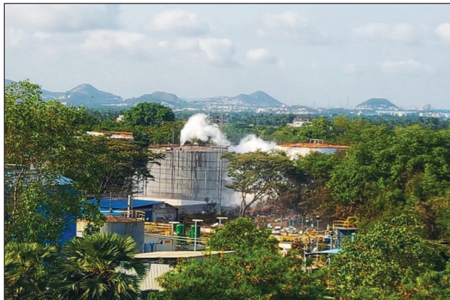
Gas leak in LG Polymers plant in Vizag.
