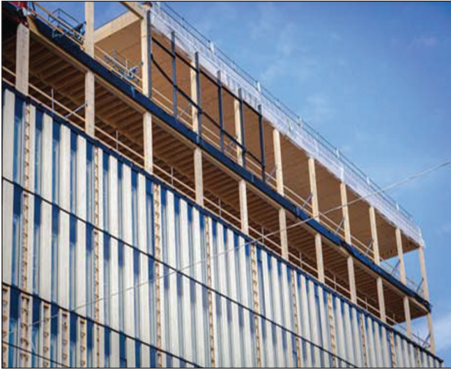
Construction of Wood City in Helsinki, Finland.
