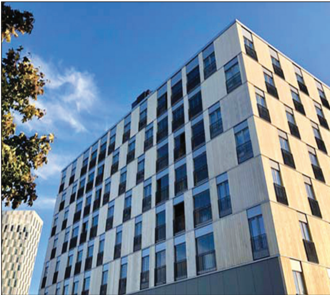
Wood City's residential in Helsinki, Finland.
