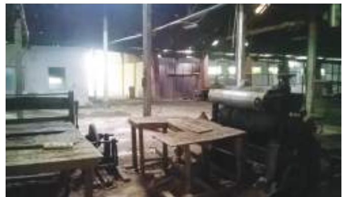
Plywood Machinery at the AR and T, Assam.
